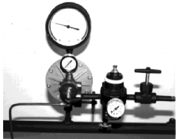
Figure 5 With Option -29; Field Pipe Niple Mounted to Piping
